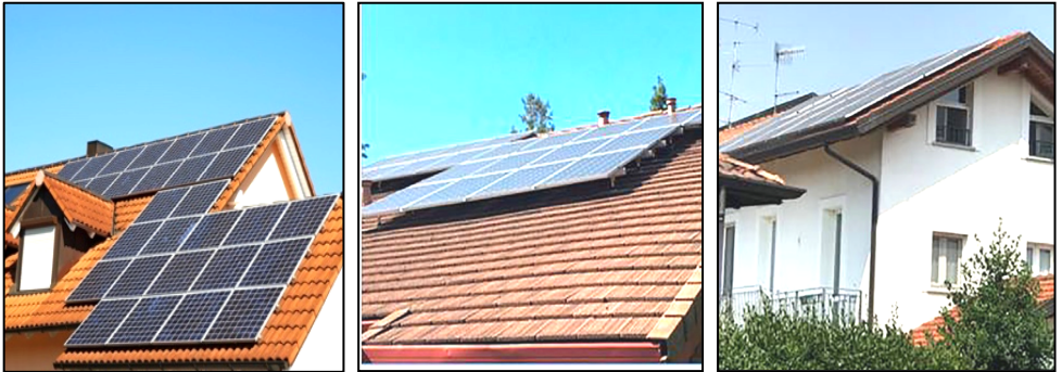
Figure 1: Examples of Rooftop PV System Installations
