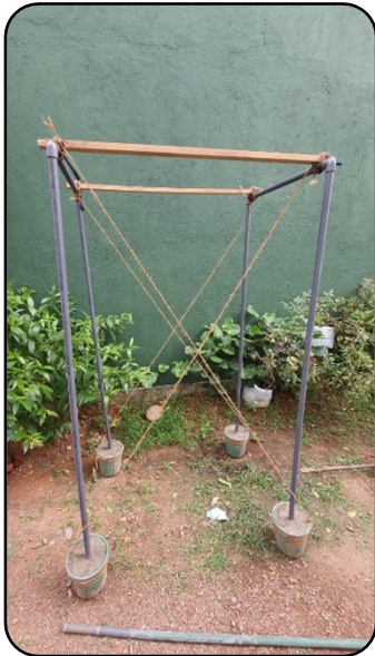
Figure 2. Greenhouse construction Step 01
