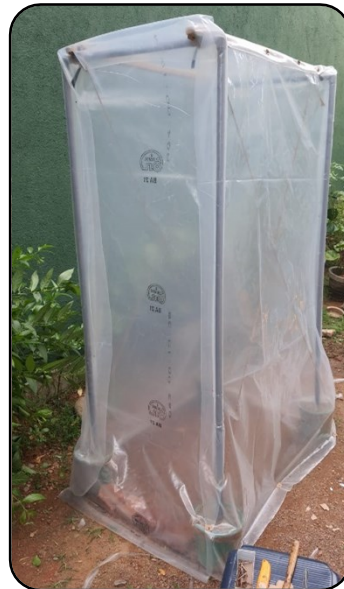
Figure 3. Greenhouse construction Step 02
