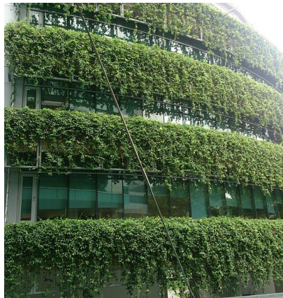
Figure 2: Vertical gardening systems
