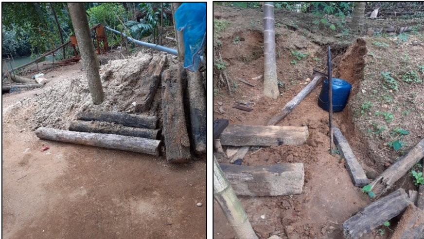
Figure 1: Stem of the Trees Use for Construction of Tunnel
