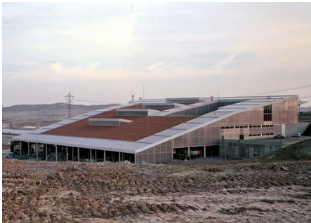
Figure 6: Recycling Plant built on a dead open dump in Madrid
