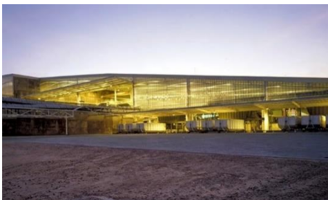
Figure 8: Building envelop finished by polycarbonate panels
